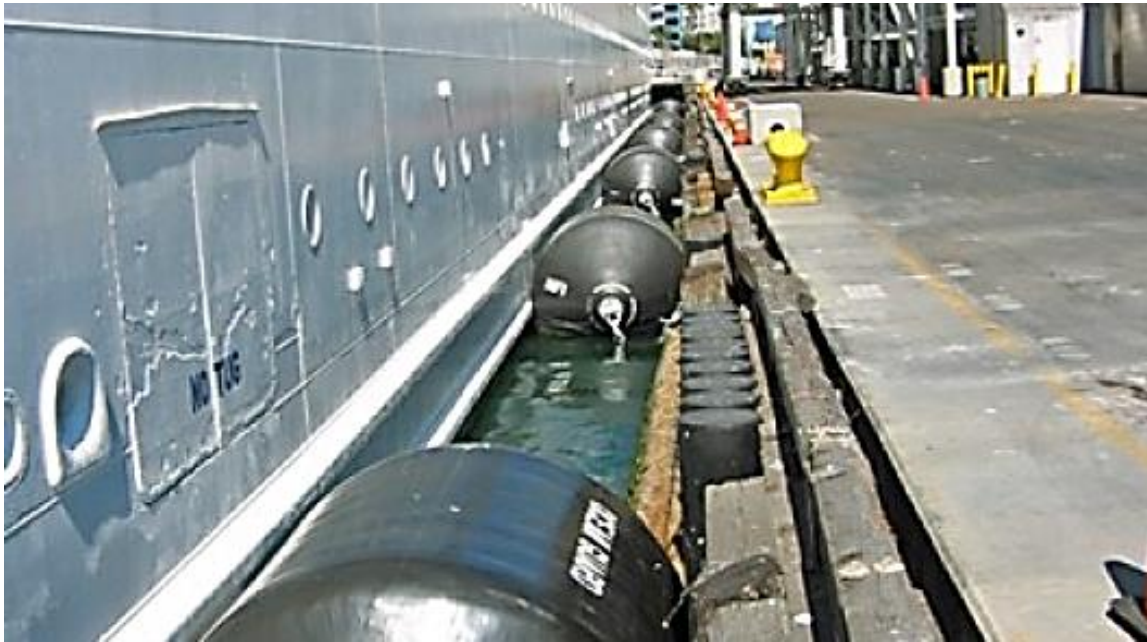
Fender Replacement at the B Street Cruise Ship Terminal
