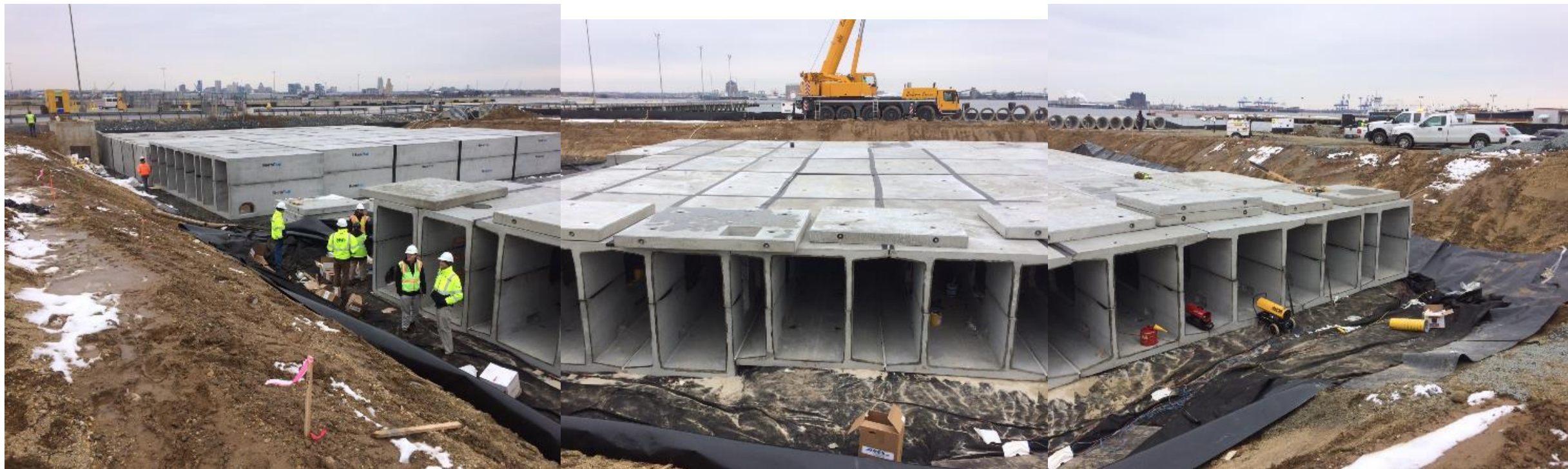
FMT Wet Basin: Large Underground Storm Water Management System, Jan. 17, 2019, (before being buried).
