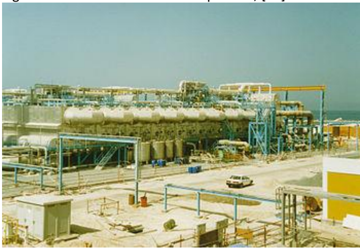
Figure 10 - MSF Desalination Plant at Jebel Ali G Station, Dubai: [28]
